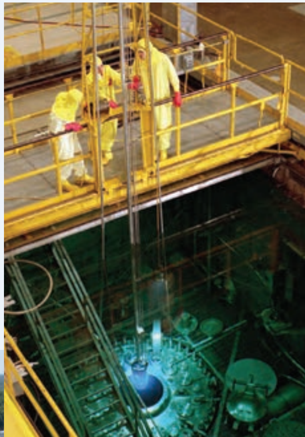
HFIR removing inner fuel element.
