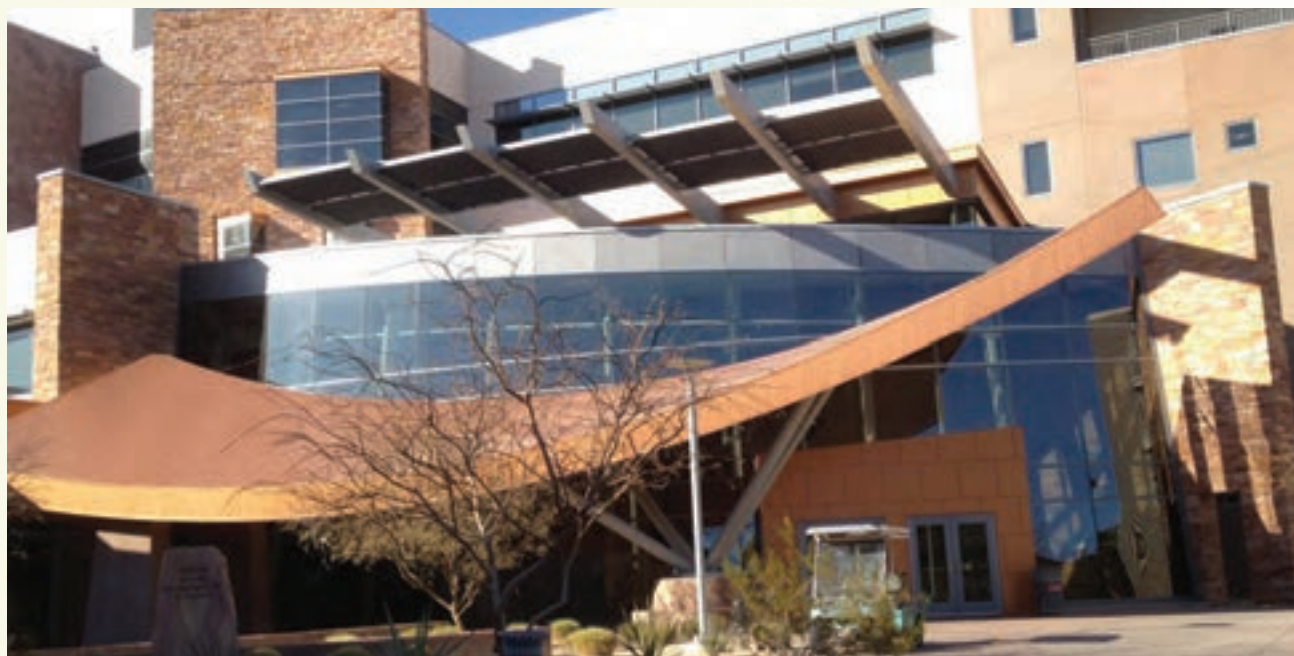
UNLV's Science and Engineering Building.
