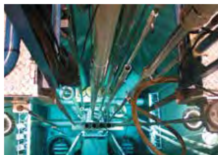
Downward view of the PULSTAR reactor pool.
