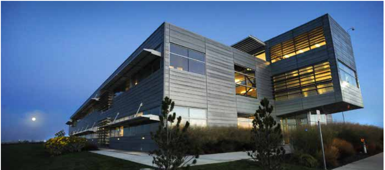
The Center for Advanced Energy Studies located on the Research and Education Campus in Idaho Falls.
